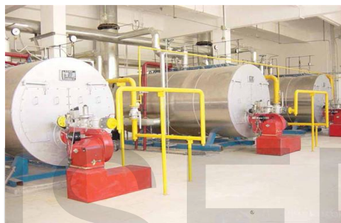
Figure.9. Combustion Chamber and Burner Management system
